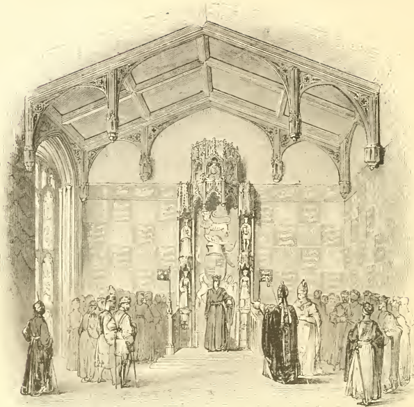
[Room of State in the Palace.]
